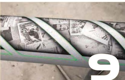
**APPLY CLEAR:** After drop shadows are applied, lay new tape over existing tape and apply two light tack coats of DC4000 clear to protect the images.
